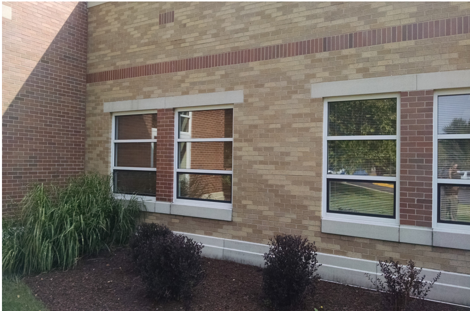
Typical exterior masonry and aluminum windows
