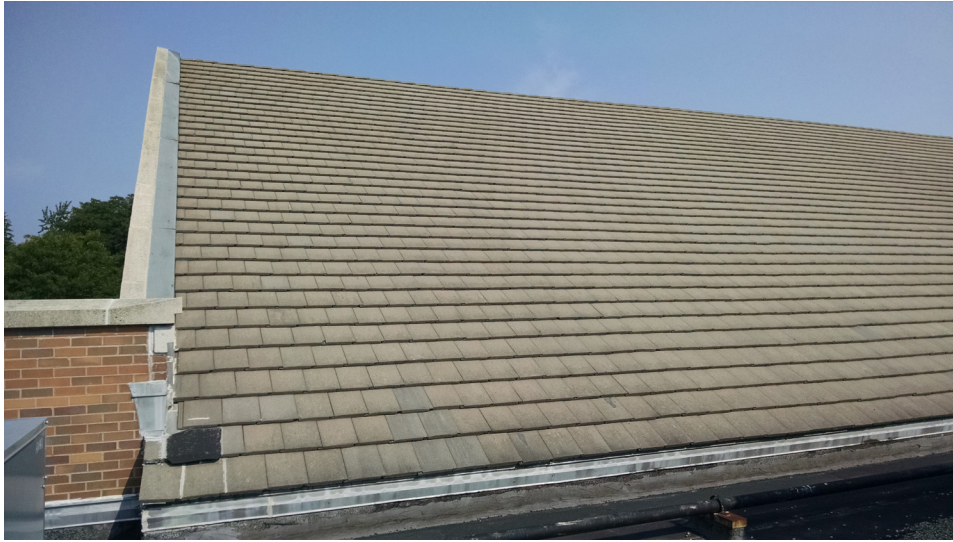
Concrete Roof Tiles at Nave
