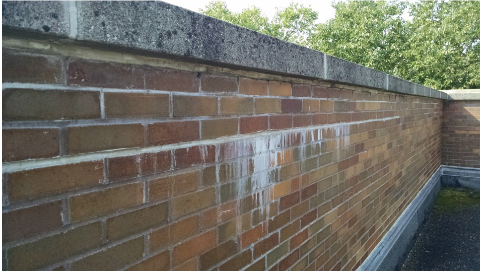
Efflorescence at Parapet Cap
