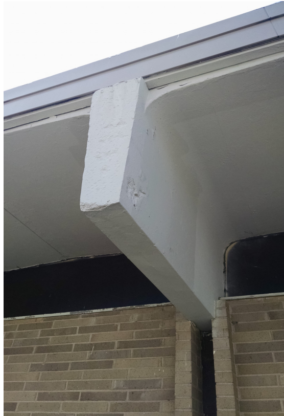
Pre-cast concrete roof members
