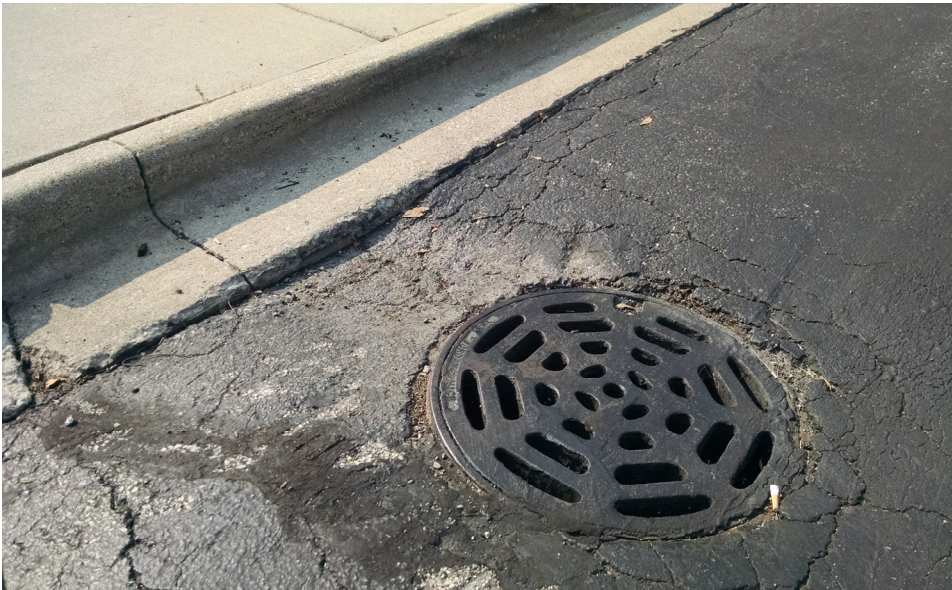
Pavement subgrade failure near catch basin
