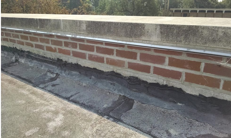
Exposed CMU at upper roof area
