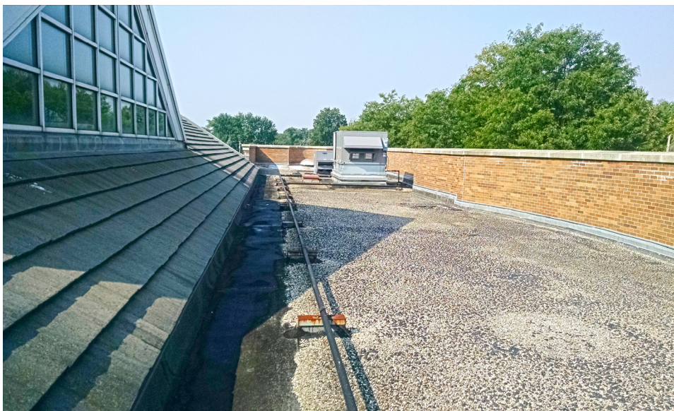
Low Slope Modified Bitumen Roof South of Nave
