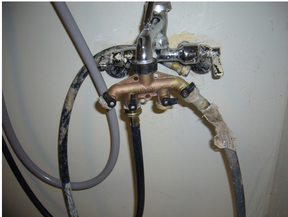
Splitter at utility sink
