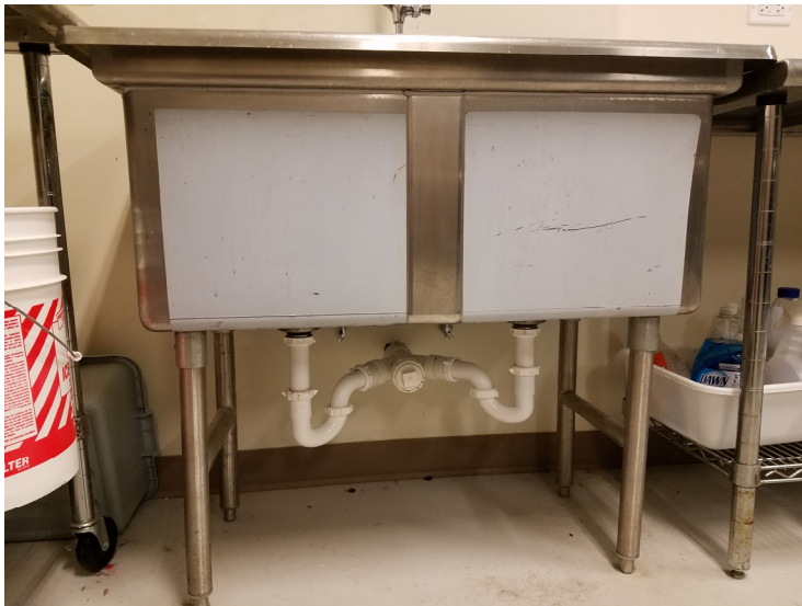
Warming Kitchen - Direct sanitary connection at double bowl sink
