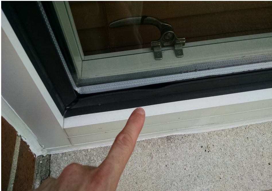
Shrinking / deformed perimeter gaskets
